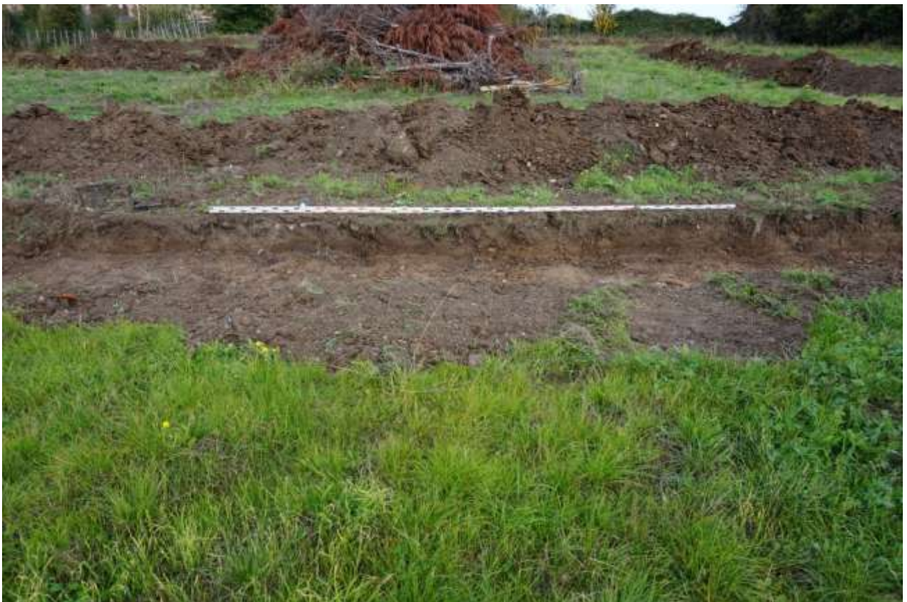
Plate 11: Looking north-west at section of trench 6.
