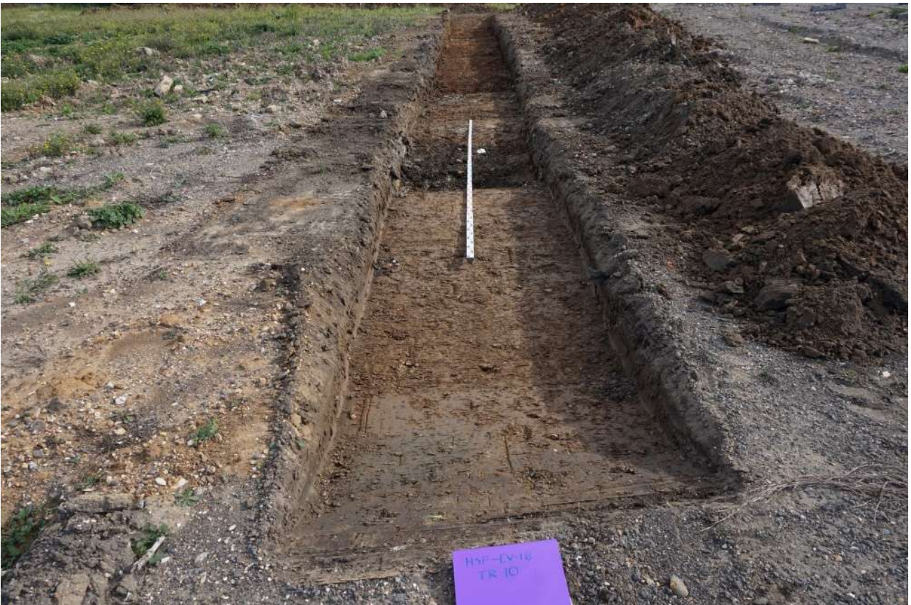
Plate 16: Looking north east at Trench 10 with machine excavated modern features.
