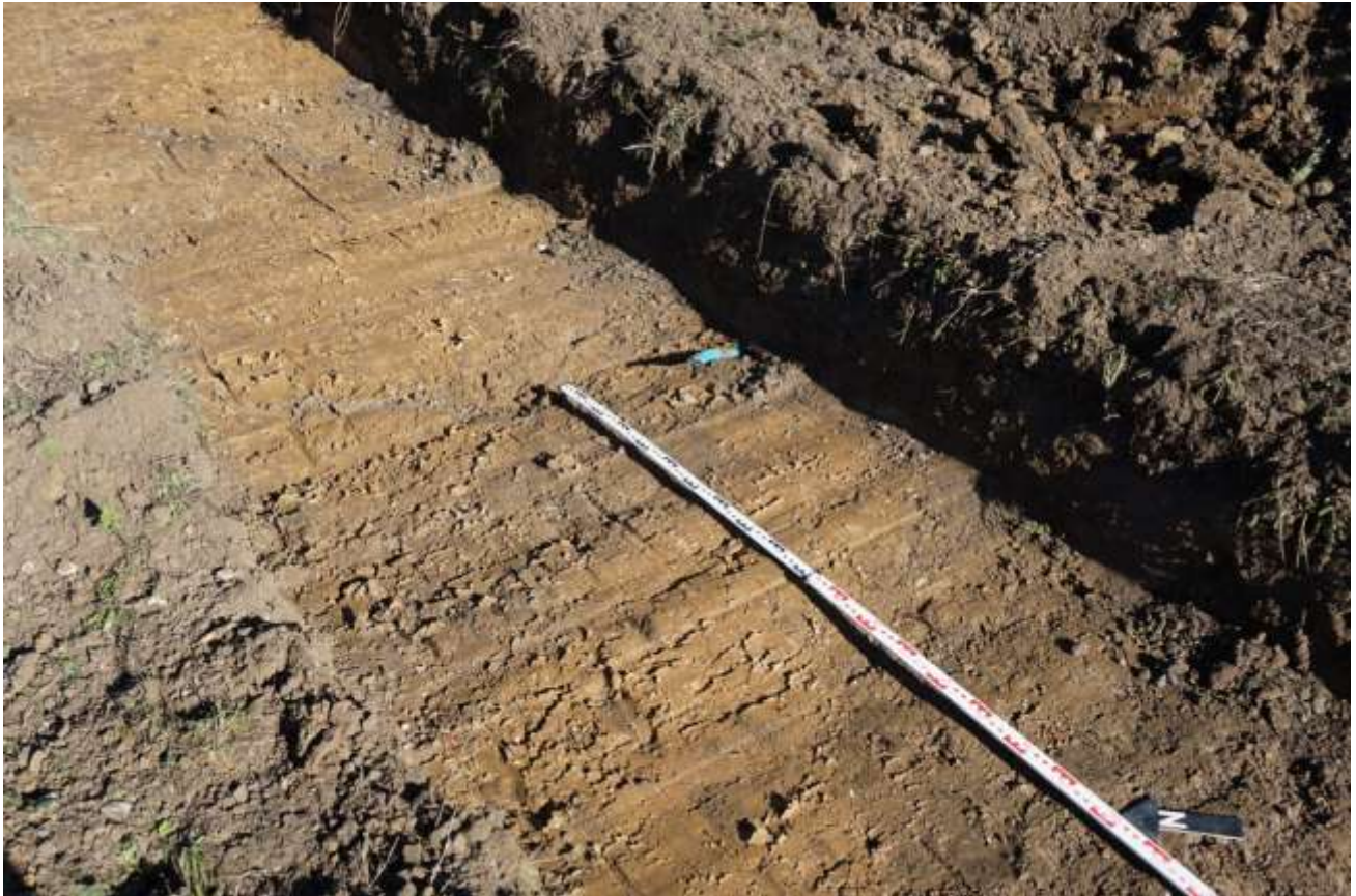
Plate 6: Looking east at plastic water pipe exposed in Trench 2
