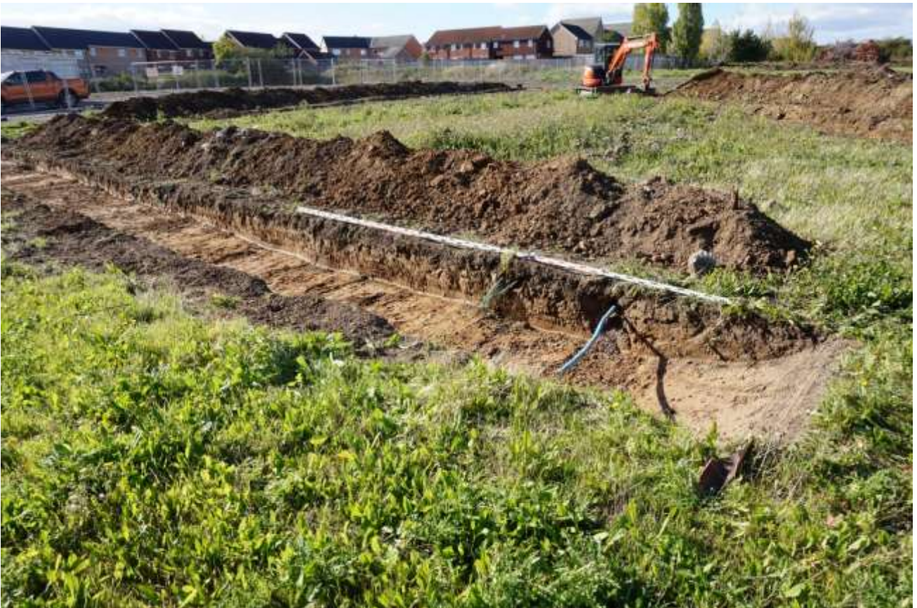
Plate 18: Looking west at Trench 12.
