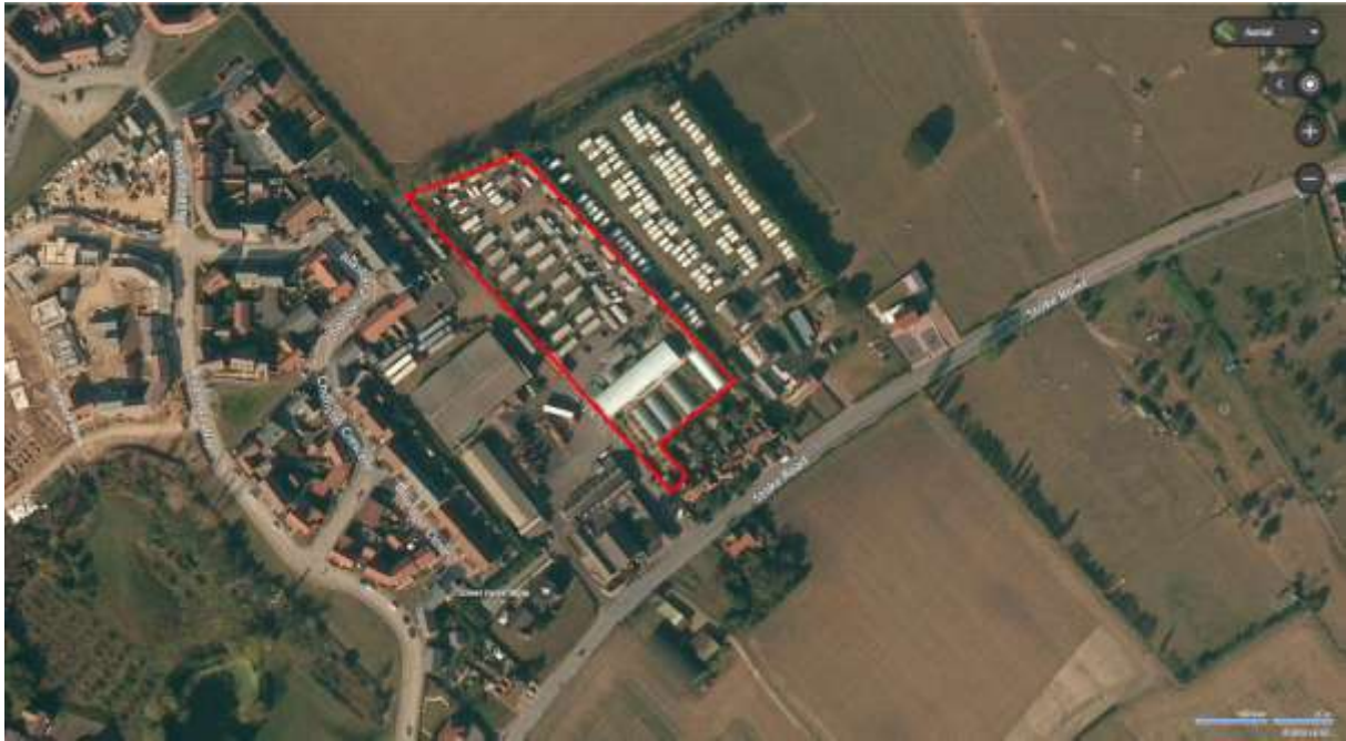
Plate 22: Aerial photograph showing the site prior demolition
