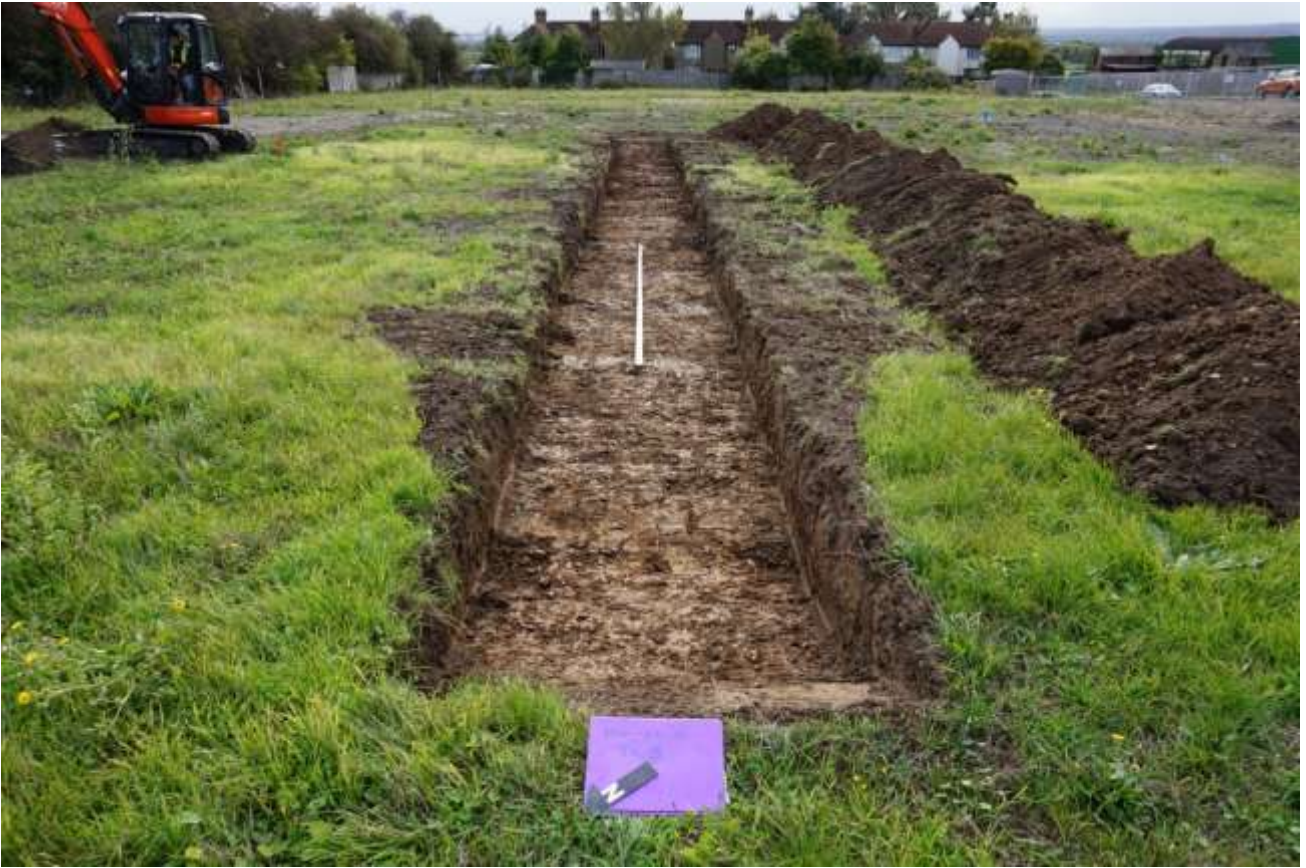
Plate 13: Looking south east at Trench 8; 5m scale.
