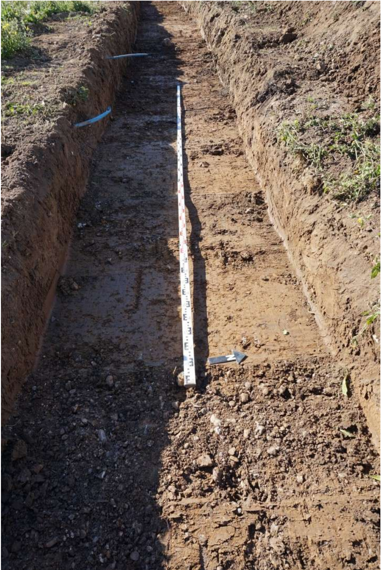
Plate 21: Looking west at Trench 14
